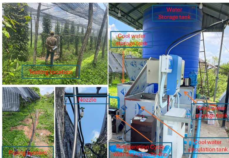
Figure 14. Photo of actual cooling system supply to testing area
