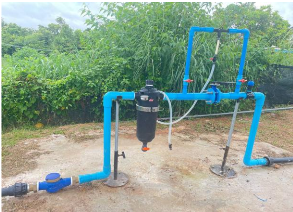
Figure 25. Drip irrigation head unit at Reaksa Farm
